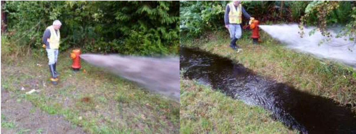
Figure 4 Distribution System Flushing
